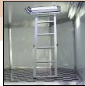
Escape Hatch with Ladder
