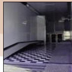
Ramp Over Wheel Wells
